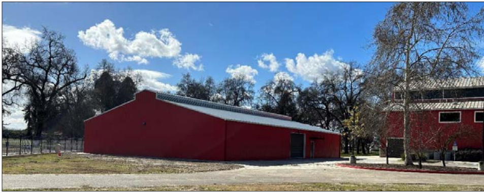
The new museum addition features restored ag equipment.
