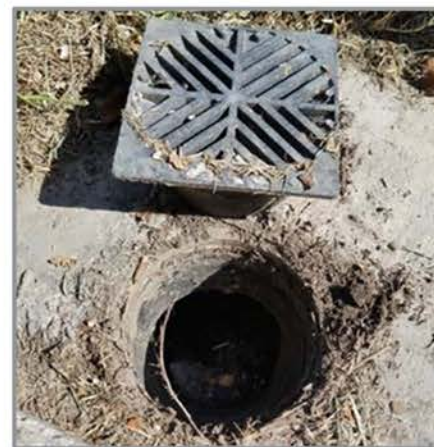
Place window screens over yard drains
