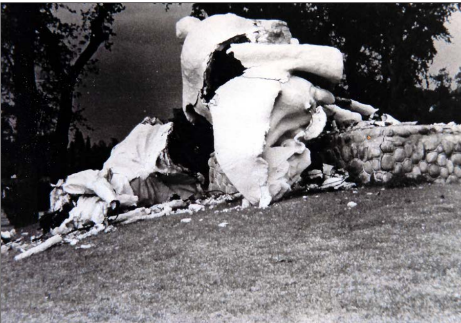
Some of the rubble after the statue collapsed in 1980
