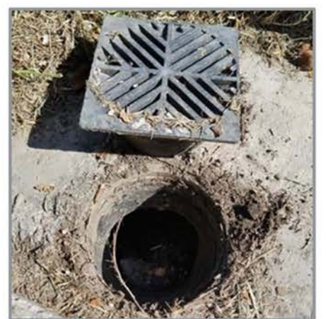
Place window screens over yard drains
