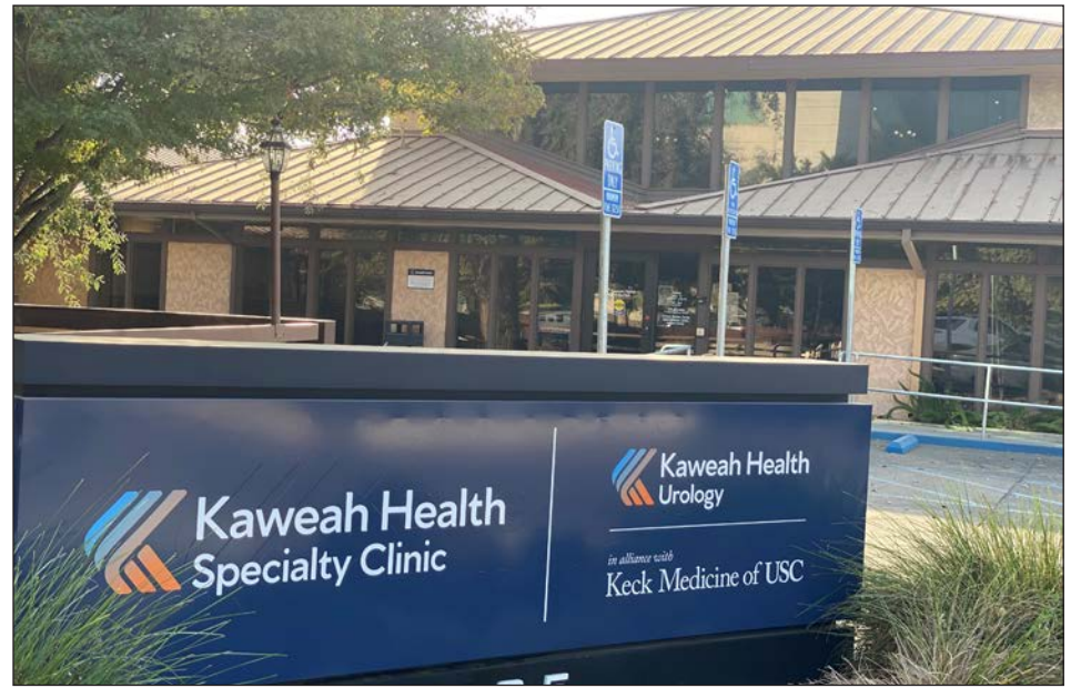
The new urology clinic is located one block west of Kaweah Health Medical Center in downtown Visalia.
