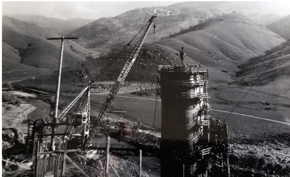
Terminus Dam under construction, circa 1961. (Photo courtesy of the History Room, Tulare County Library)
